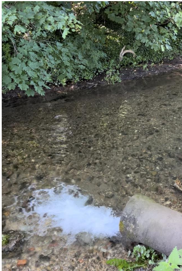
Figure 25 Water flowing from the blow well into the Laceby Beck.
