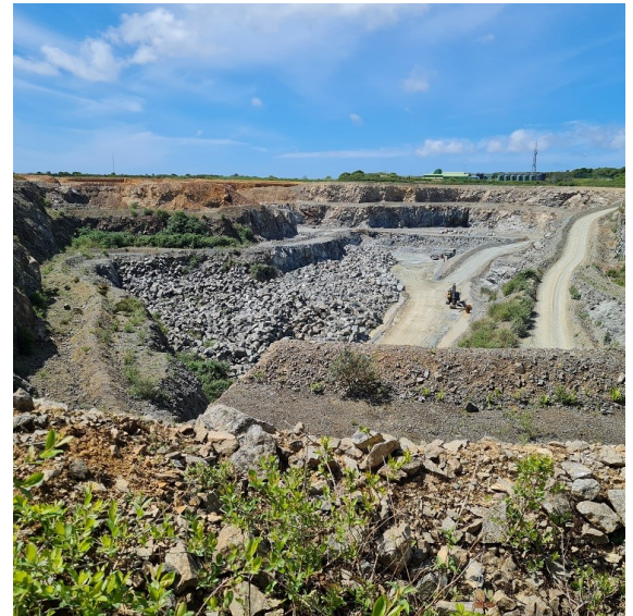
Fig. 5 view of quarry from haul road
