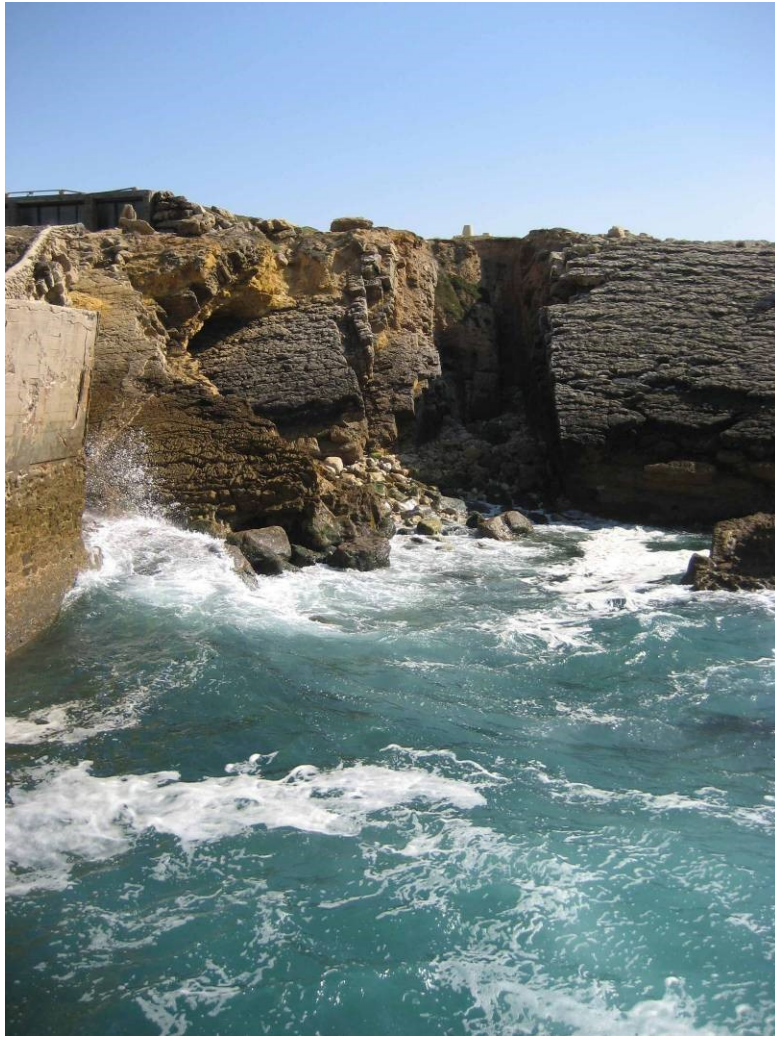
Fig 3, Eroded dyke in the inlet referred to in Stop 3
