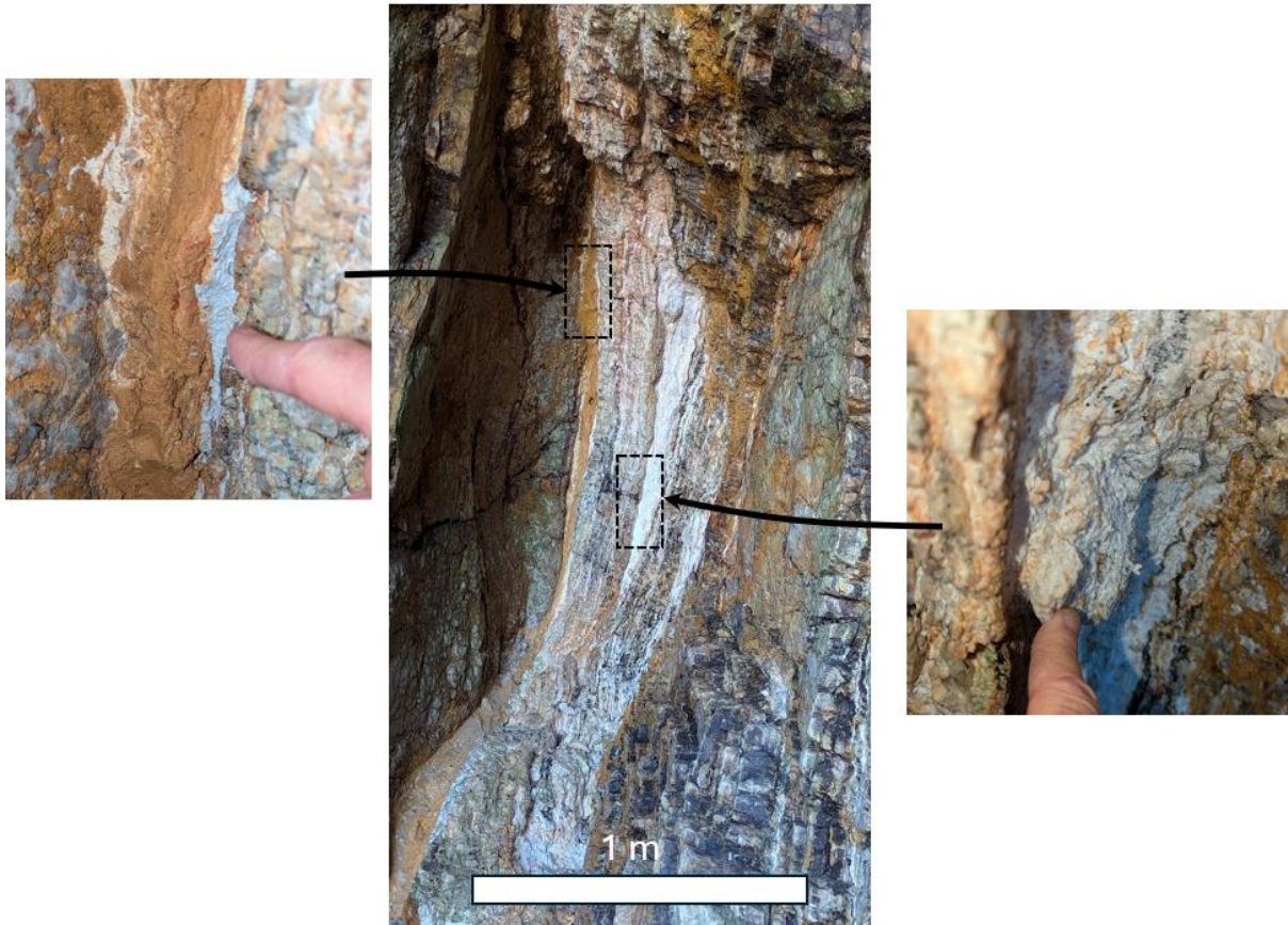
Figure 24 Internal structure of Carn Clew fault zone and mineralisation, with orange clay (left) and white sandy clay beds (right).
